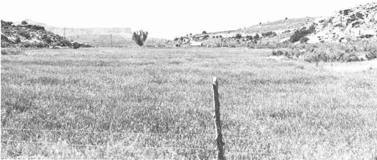
Figure 58. Mud Creek Damsite. View looking upstream at Mud Creek Damsite. Dam location is just downstream from building in center of photo. C-1244-406-16
