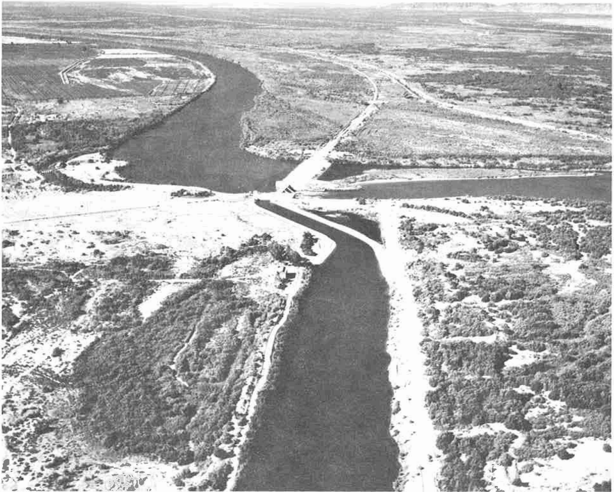
Figure 29. View showing the Palo Verde Diversion Dam on the Colorado River and the headworks of the District's main canal. P385-300-5769 NA
