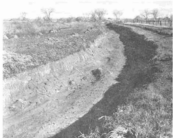
Figure 15. Typical section of an unlined canal in the Grand Valley area. P1244-427-44 NA
