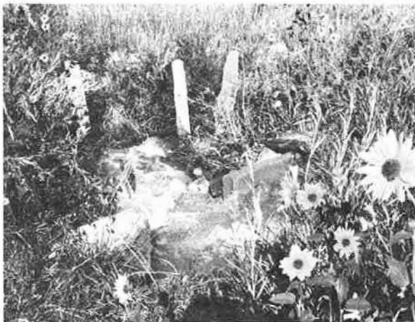
Figure 36. Diversion structure showing how ditches are infested with weeds and difficulty in obtaining measurement of water application.
